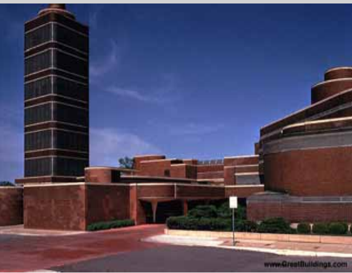
JOHNSON WAX BUILDING FRANK LLOYD WRIGHT 1944
